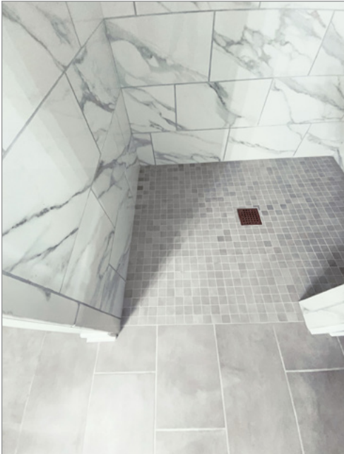
Not only are zero-threshold (curbless) showers safer and more accessible, but they are easier to clean, and the seamless look can make bathrooms look larger. Photo courtesy of Paragon Building Group.
