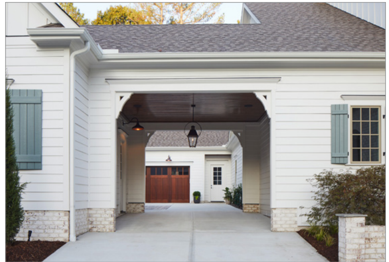
The adaptations Paragon includes in its projects range from wider doorways and larger turning radiuses around cabinetry to shafts for future elevators and backfilling the garage to create a barrier-free entry to the house. Photo courtesy of Paragon Building Group.
