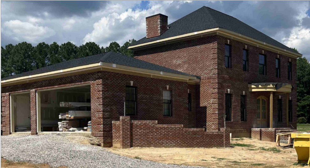
One approach to creating a barrier-free entry with no steps into the house is to backfill the garage to create a subtle change in grade from the driveway; the garage slab is lifted a bit higher and backfilled to achieve a zero transition as you enter the home. Photo courtesy of Paragon Building Group.
